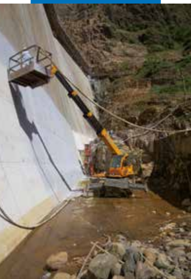
Waterproof coating on a dam
