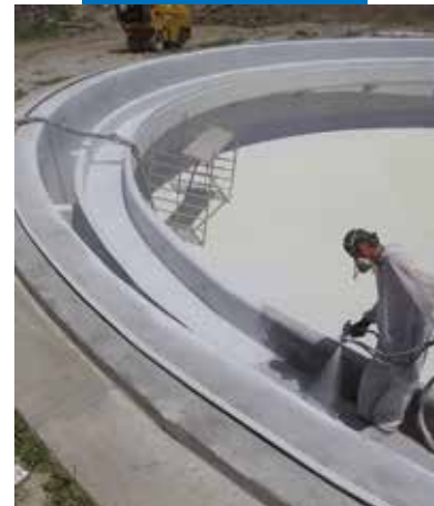
Application of Purtop 1000 onto industrial storage tanks
