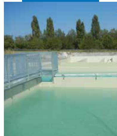
Storage tanks waterproofed with Purtop 1000
